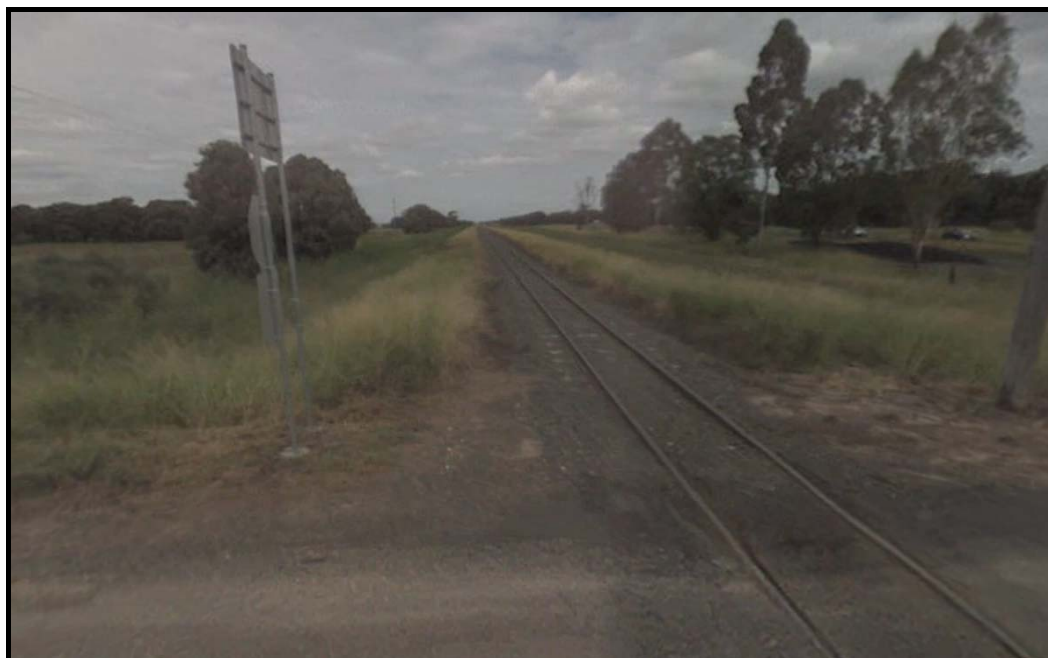
FIGURE 16.4 RAIL LINE NEAR THE STUDY AREA
